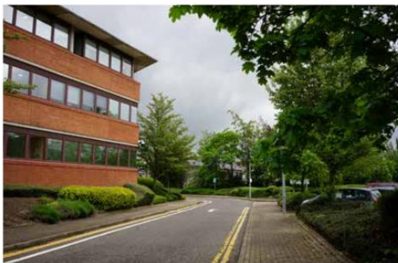
5. Southern Service Road
