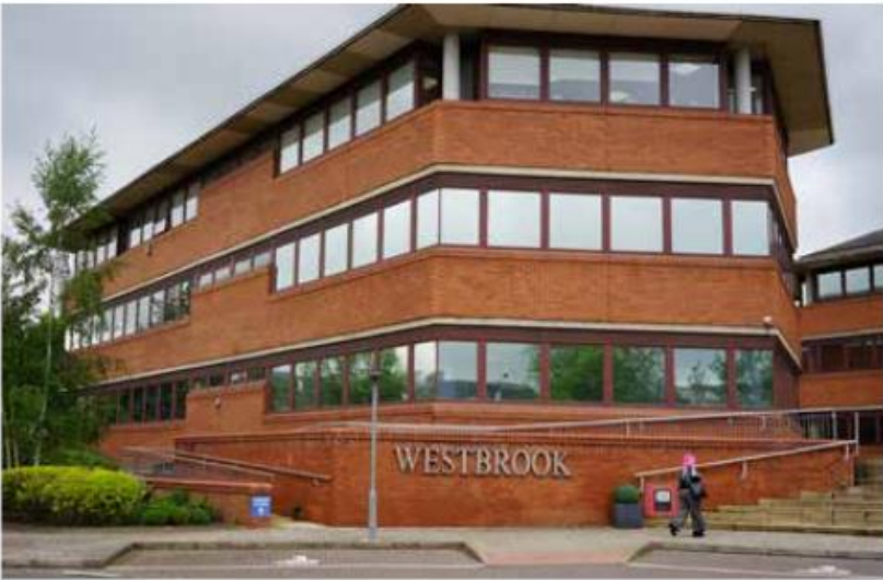
2. Existing ramp access and signage
