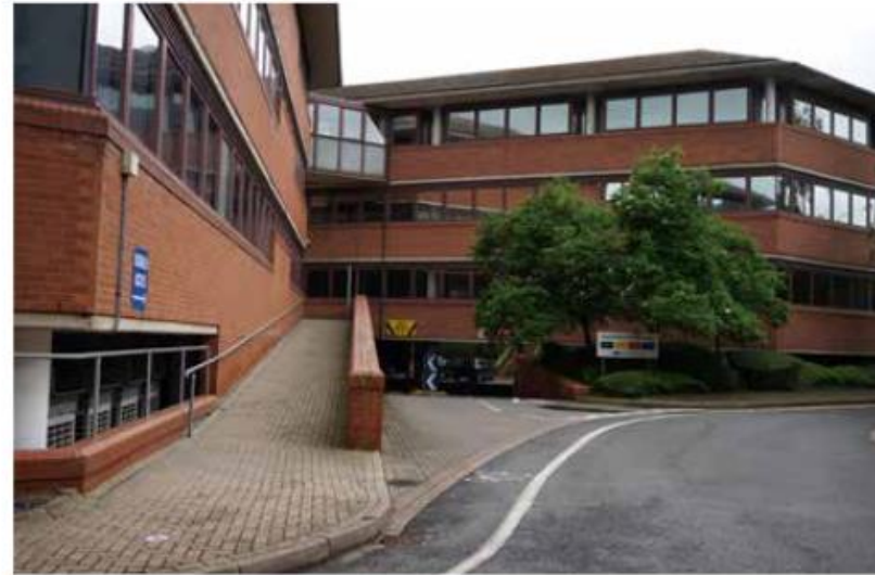
3. View into the undercroft parking and adjacent ramp access to ground floor
