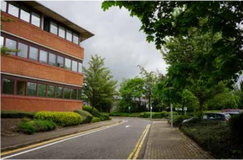
5. Southern Service Road
